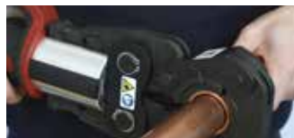
3. Complete the joint with the press tool
