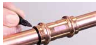
7B. Alternatively insert tube to tube stop and mark
