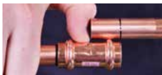
7B. Check the depth mark
