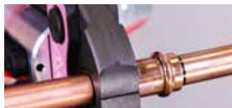
2. Complete the joint with the approved tool. Press once only
