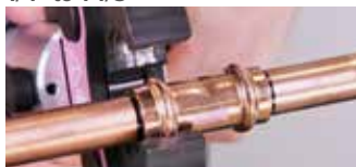
1. Align jaws squarely on the fitting
