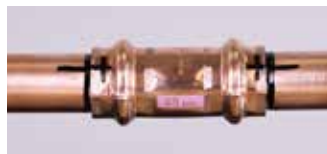
3. Mark the completed joint
