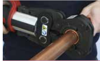
3. Complete the joint with the press tool
