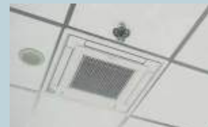
Integrates easily into the 600 x 600 ceiling tile, enabling lights, speakers and sprinklers to be installed in adjoining tiles
