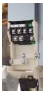
Bigger working space for wiring connection.
